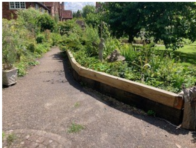
G: H: & J: Illustrating banks which were created from the earth removed when making the new pathway. By creating the banks the level of the plants is higher and brings them into closer to the field of visitors especially those in wheelchairs
